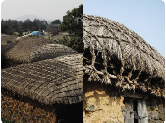
A traditional roof designed to withstand the high winds of Jeju Island. The straw roof is tied down and pitched at a low, curved angle.
