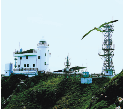
Dokdo Lighthouse First set up in August 1954; extension of facilities and introduction of manned service in December 1998; 1 Unit (lighting up to 25 miles; Staff: 3; Height: 15m; Area: 161 m 2 ; 2 Diesel Generator(75 kW); Sunlight Generator (15 kW)
