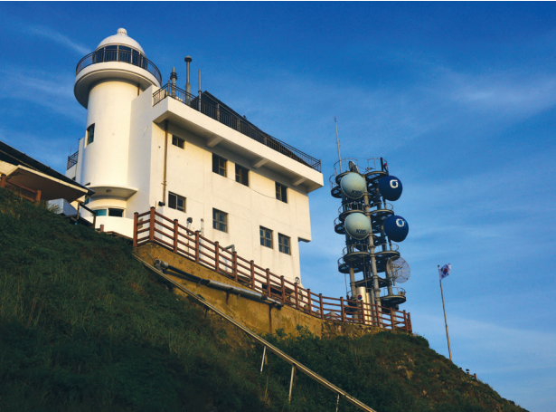
Dokdo Lighthouse First set up in August 1954; extension of facilities and introduction of manned service in December 1998; 1 Unit (lighting up to 25 miles; Staff: 3; Height: 15m; Area: 161 m 2 ; 2 Diesel Generator(75 kW); Sunlight Generator (15 kW)
